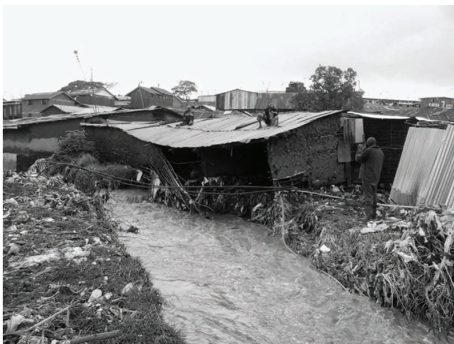
Figure 3. High waters and flood damage on the Ngong River in the Andolo area of Kibera after heavy rains on 12 May 2015. Photograph by Pascal Kipkemboi (KDI)
