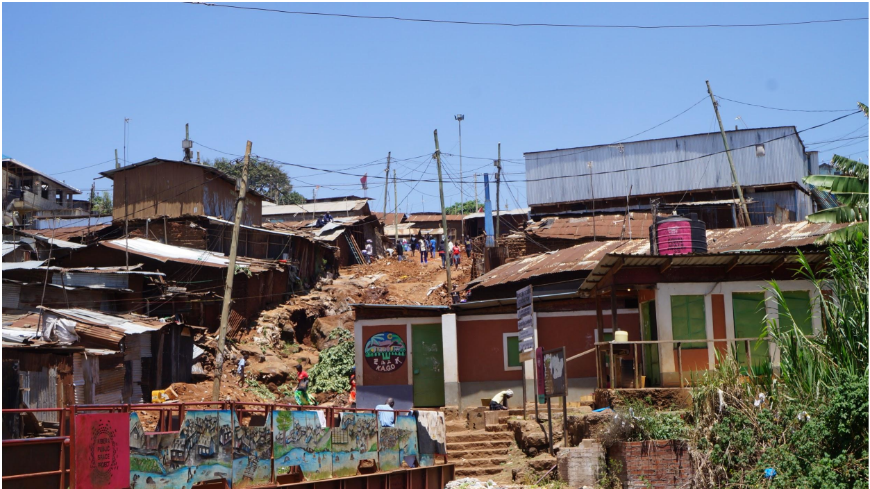
Photo 2: Dead end access road in Gatwekera Village with 34% gradient (KDI, 2021)
